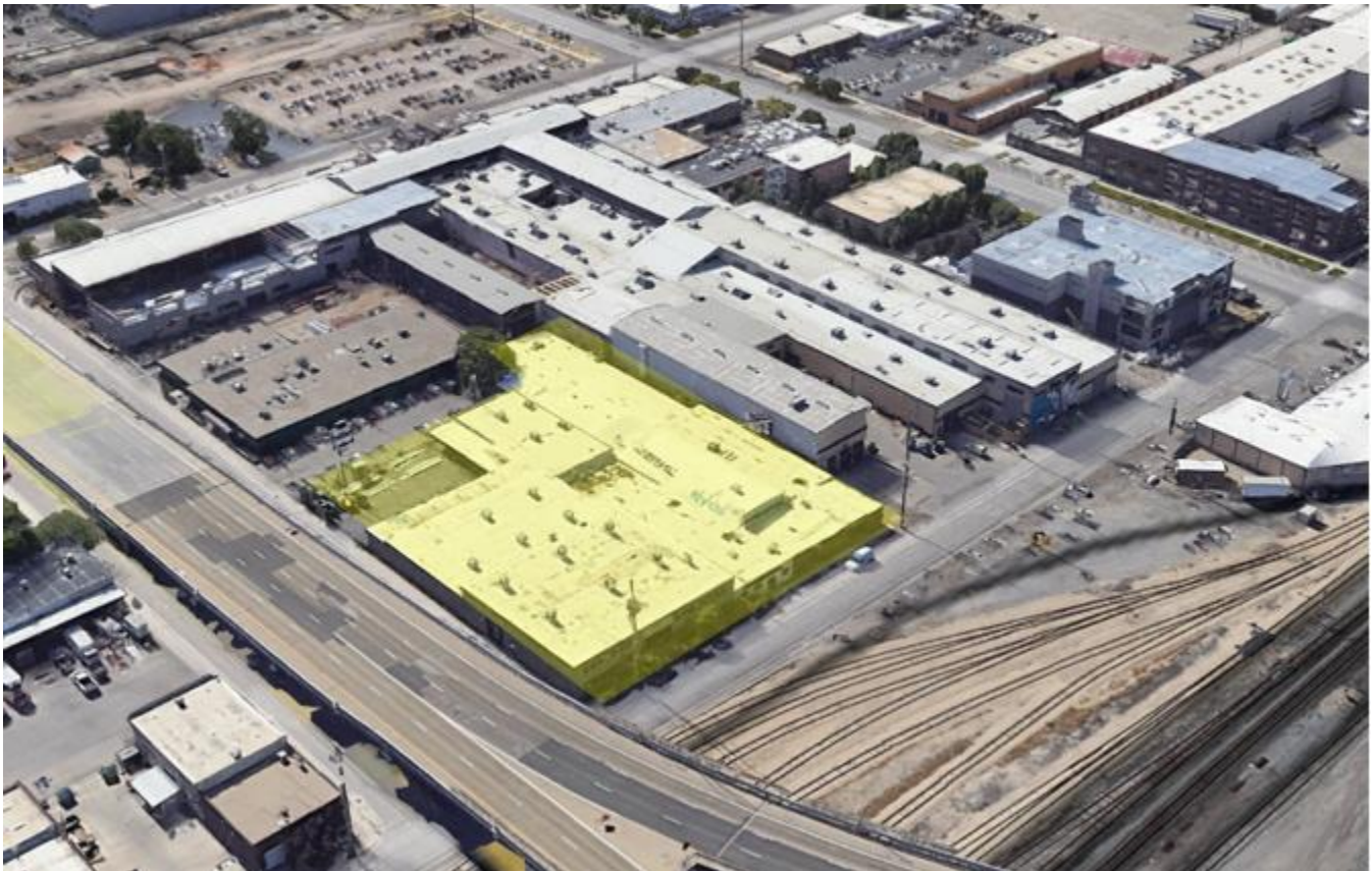
Subject Property from northwest looking southeast
